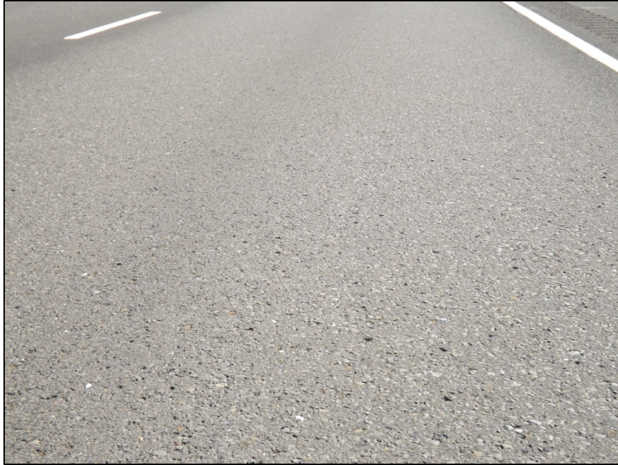
Figure 28 HMA Surface Texture at 39-Month Revisit in Walla Walla, WA
