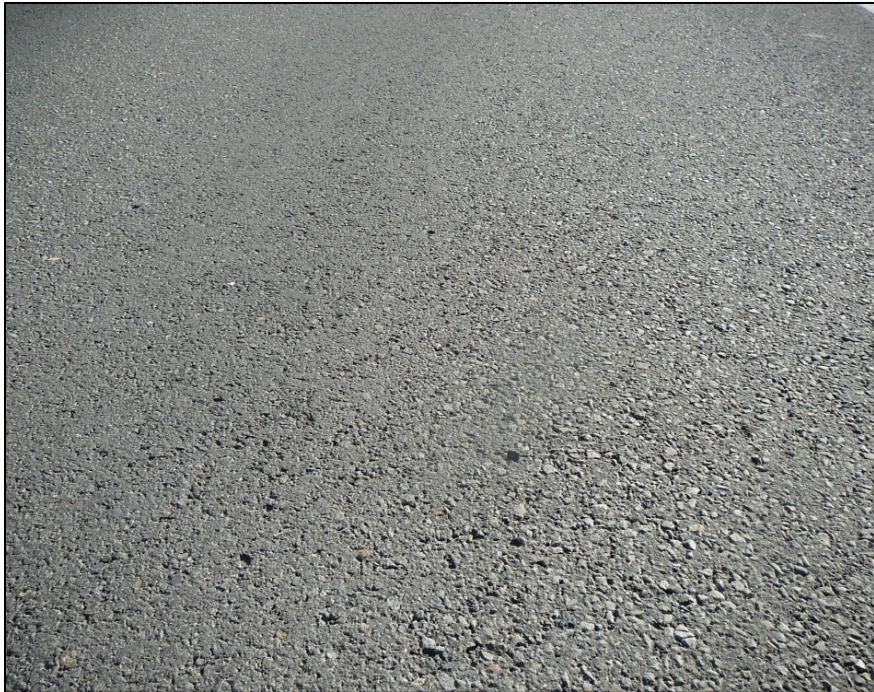
Figure 25 HMA Surface Texture at 13-Month Revisit in Walla Walla, WA
