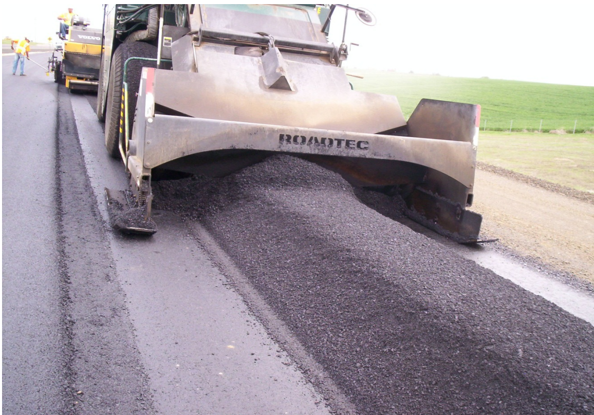
Figure 6 Material Transfer Device and Windrow
