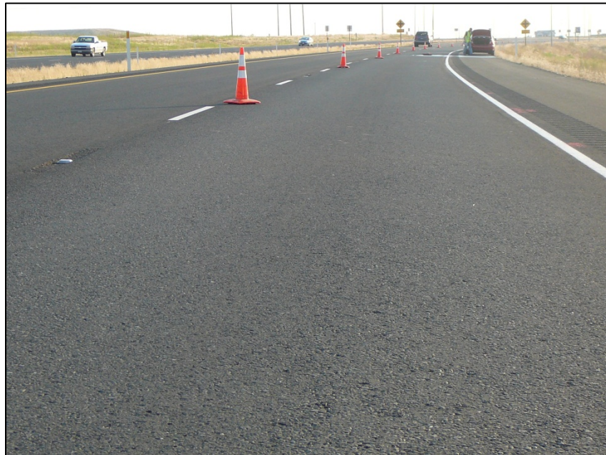
Figure 27 Example of Surface Texture at 27-Month Revisit in Walla Walla, WA
