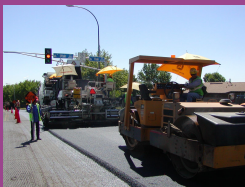
Final lift being placed
