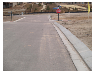
Placement of HMA to top edge of curb.
