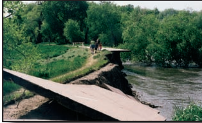
Concrete trail collapsed on Poudre River near Ft. Collins.
