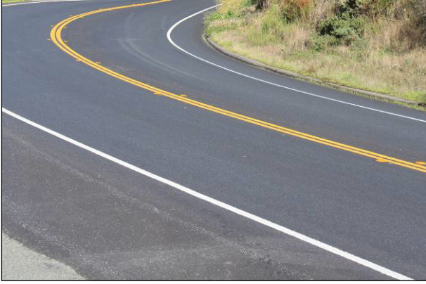
Figure 5.7: Gencor Ultrafoam 05/2011: General view.
