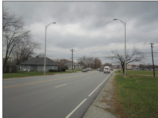
Figure 4: WMA 11/2010: General view
