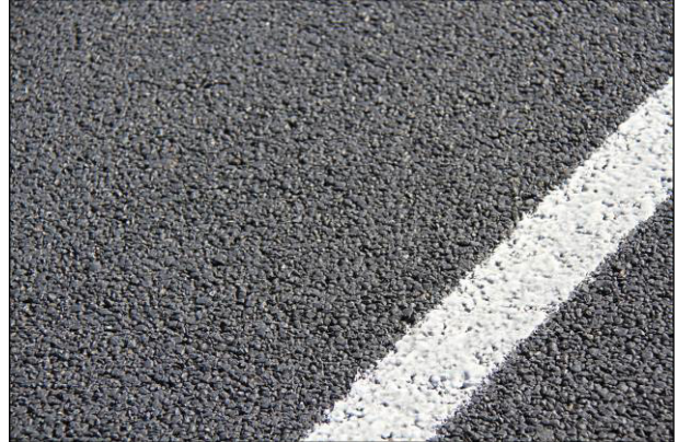
Figure 5.8: Gencor Ultrafoam 05/2011: Close-up view.
