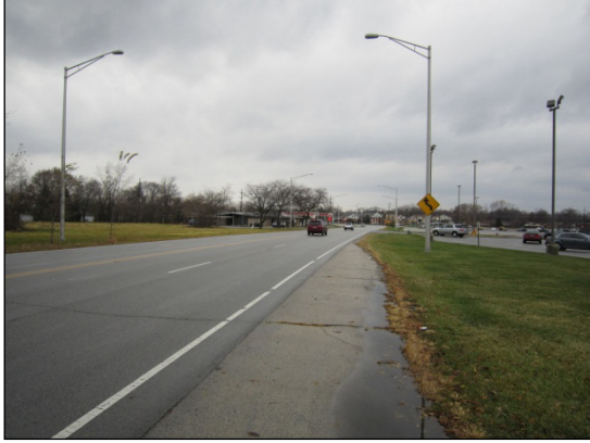
Figure 7: WMA 11/2010: Reflective crack
