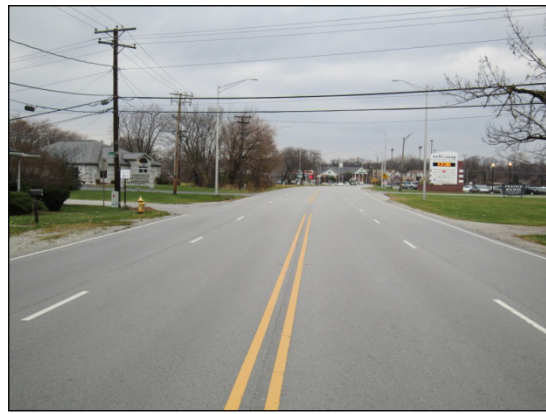
Figure 10: WMA 11/2010: General view
