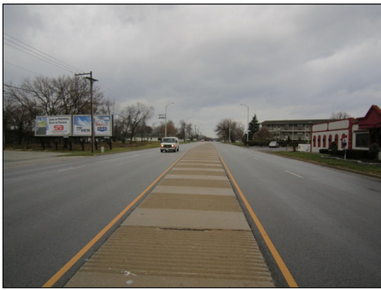
Figure 9: WMA 11/2008: General view
