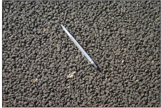
Figure 5.2: Control 06/2010: Close-up view.
