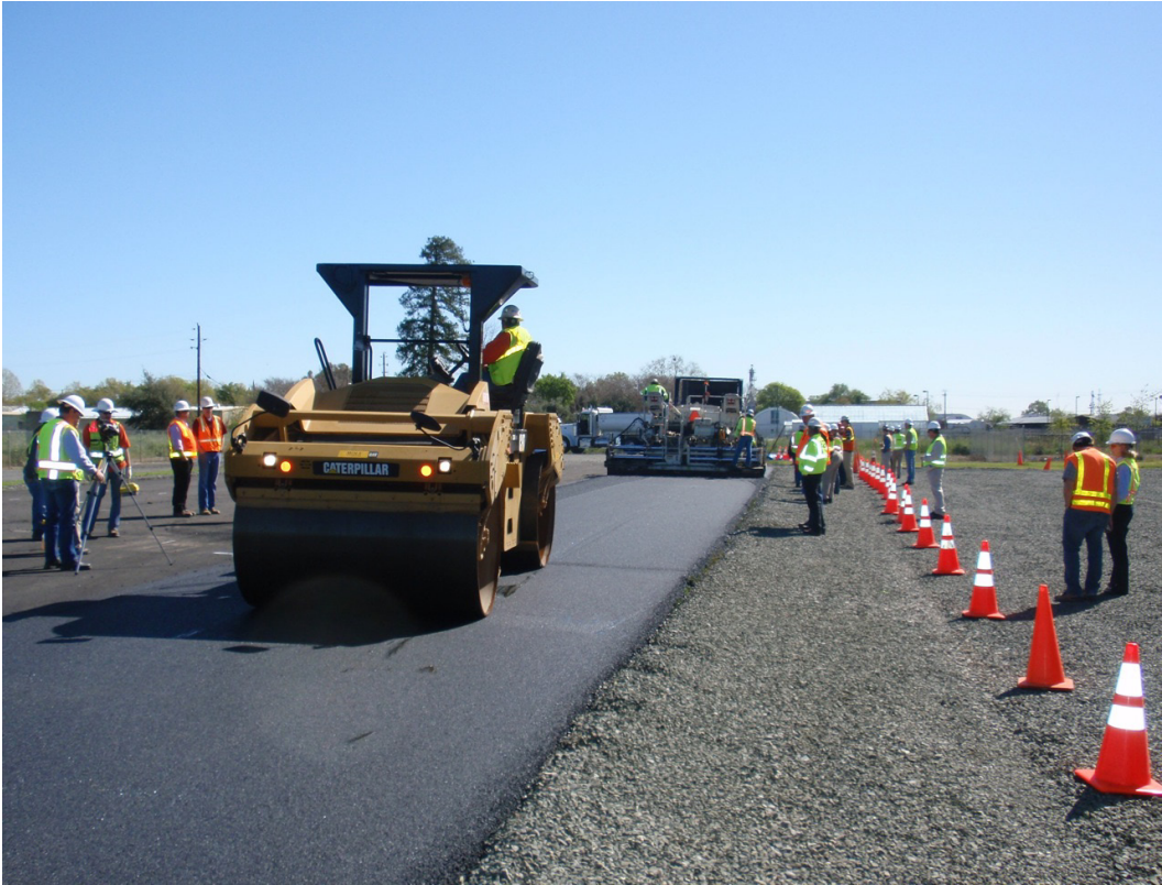
Paving WMA Rubber mix
