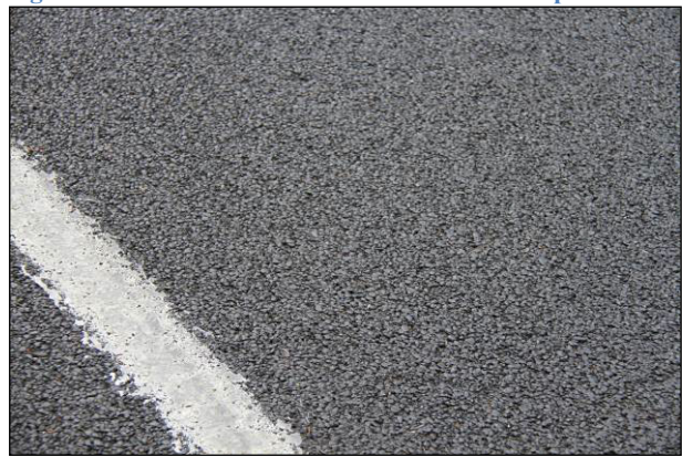
Figure 5.6: Control 05/2011: Close-up view.
