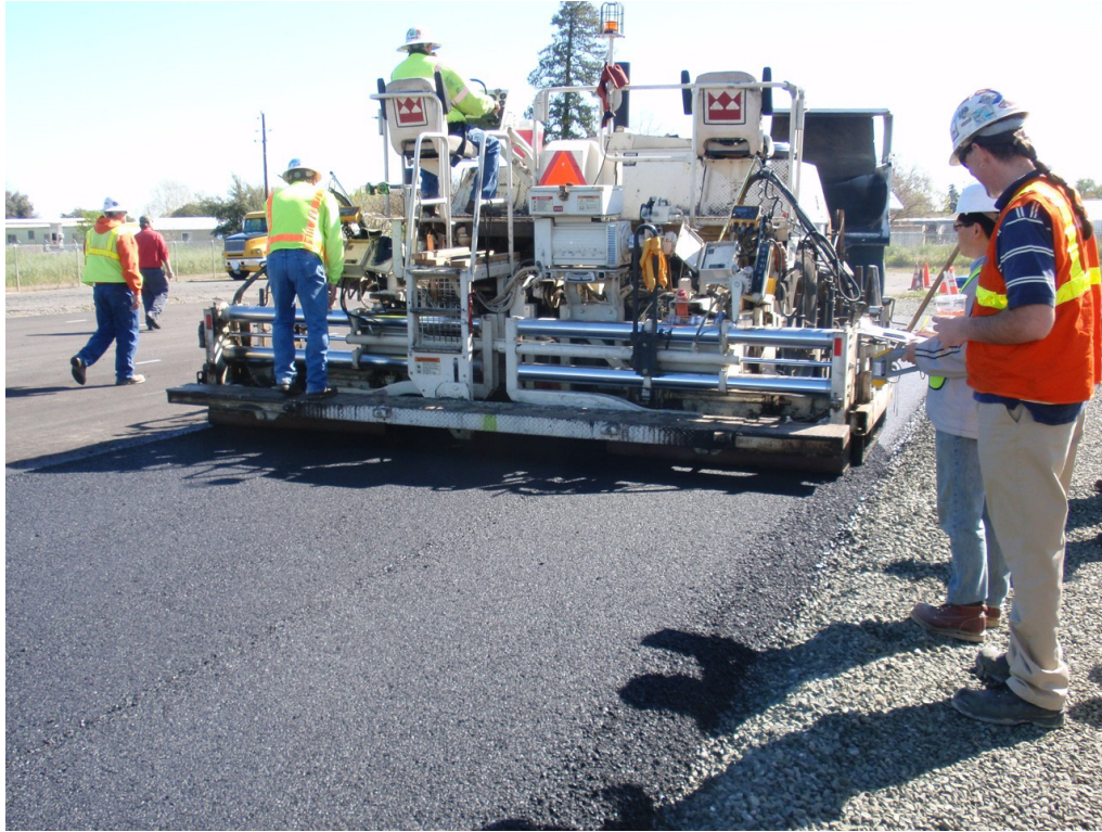
Paving WMA Rubber mix
