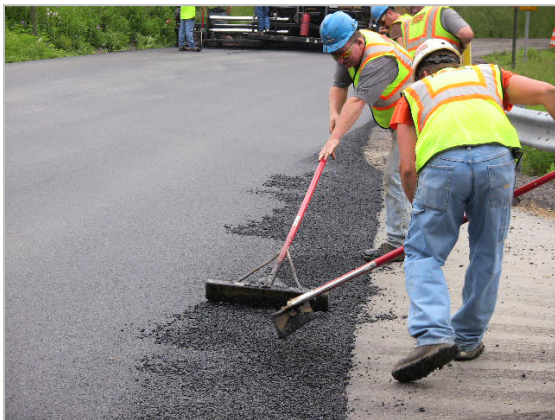
Figure 5: WMA Placed June 2009
