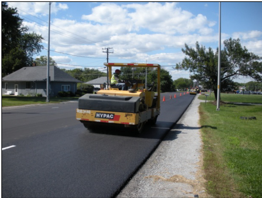
Figure 3: WMA 09/2008: General view
