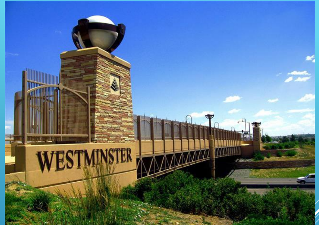
Railings & Architectural Fencing 44 Locations, 12 Bridges over State Highways
