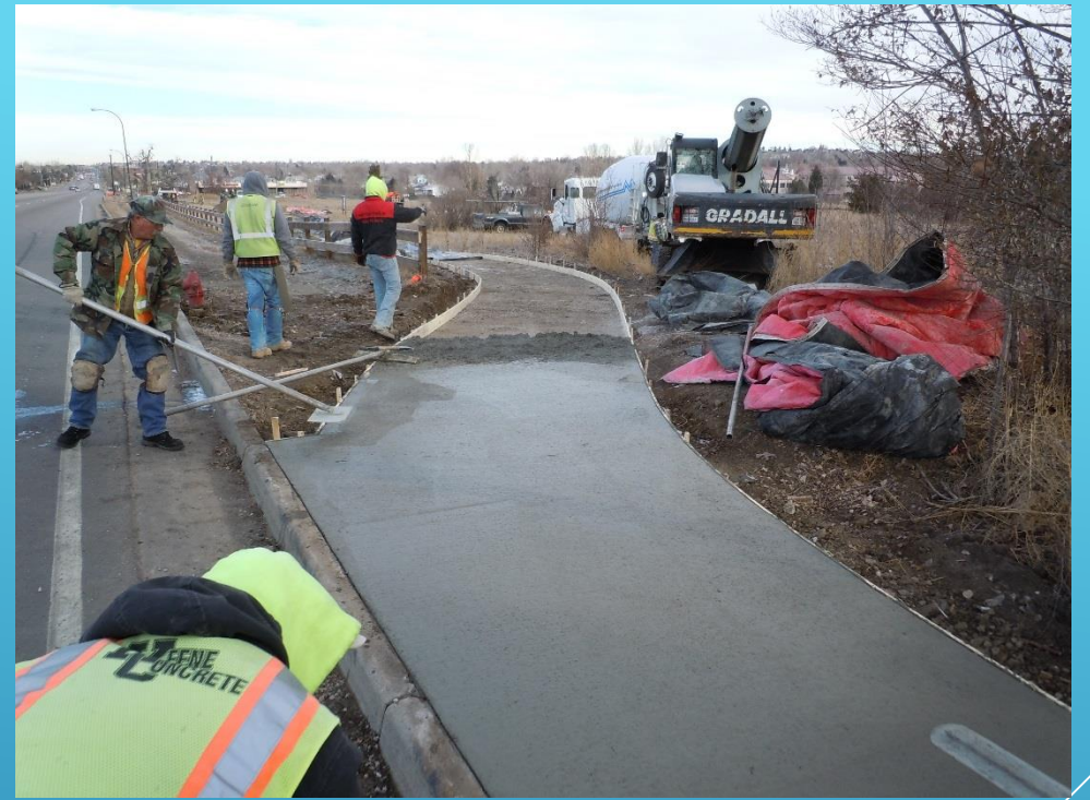
Concrete Replacement and ADA requirements
