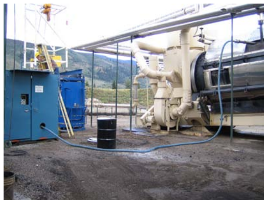
Figure 8 Feeding Sasobit through Fiber Feed Line
