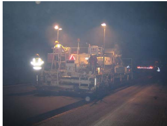
Figure 3 Visible Smoke and Fumes during HMA Placement
