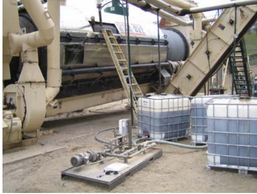
Figure 10 Adding Evotherm DAT Additive with Binder into Mixing Drum
