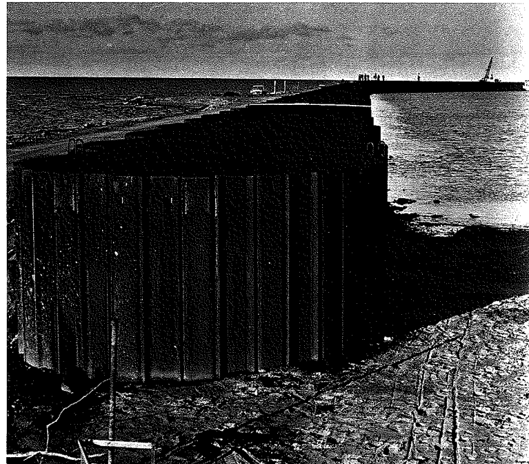
FIGURE VII-4. Asphalt-capped cellular breakwater, Port Austin, Michigan.
