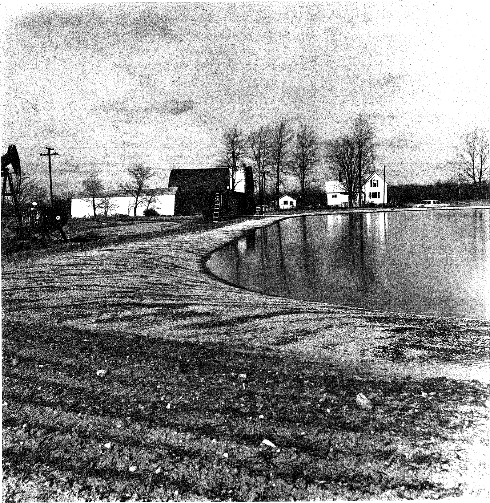
FIGURE VIII-1. Asphalt-lined brine-storage reservoir, Lapeer County, Michigan.
