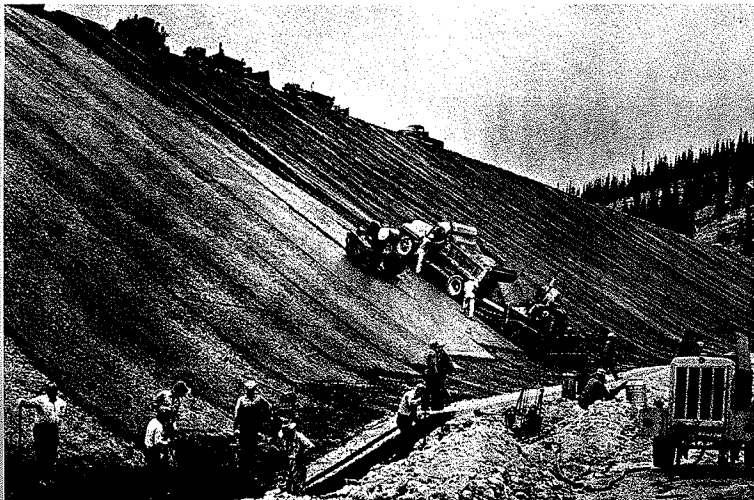
FIGURE IV-15. Paving operations, Montgomery Dam, Colorado.
