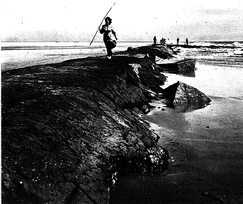
FIGURE VII-3. Galveston Jetty after fifteen years of service.
