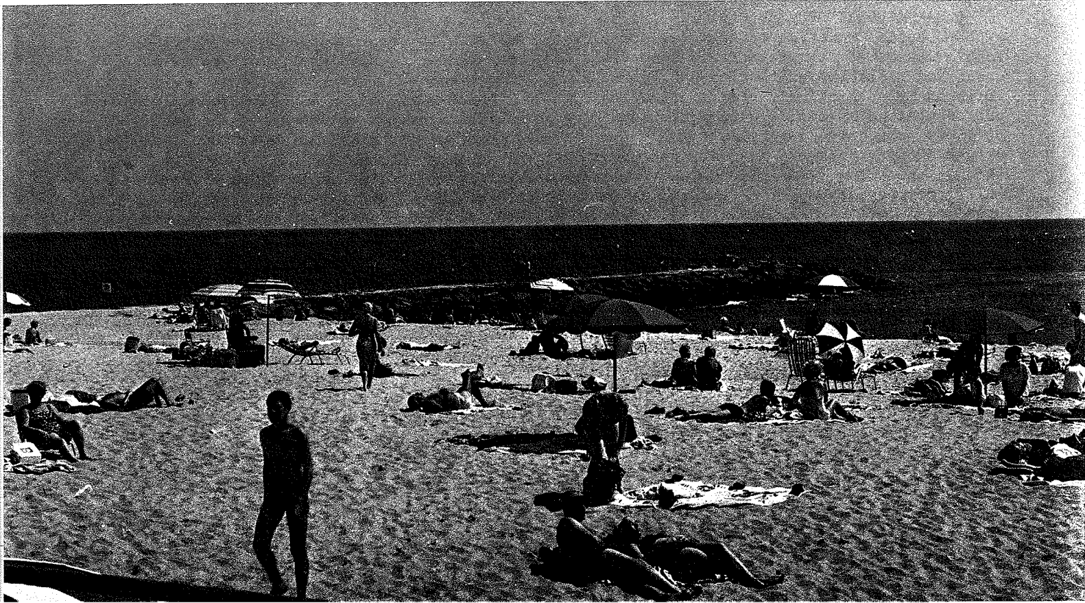
FIGURE VII-1. Asphalt jetty affords excellent protection to sandy beach, Asbury Park, New Jersey.
