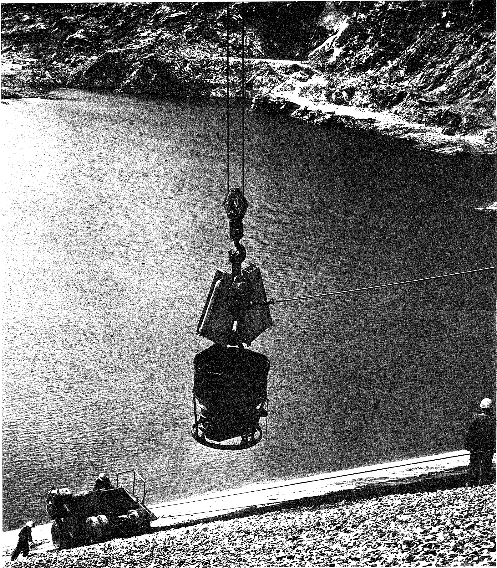
FIGURE III-1. Asphalt hot-mix being lowered to paver on Homestake Dam, Colorado.
