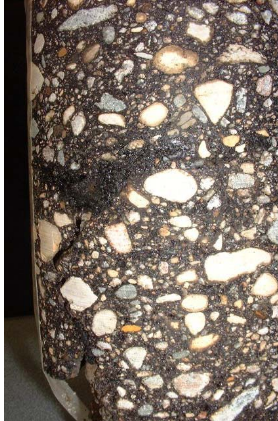
Figure 6.14. Core extracted from station 20+00 at the overlay project in Lyon County.
