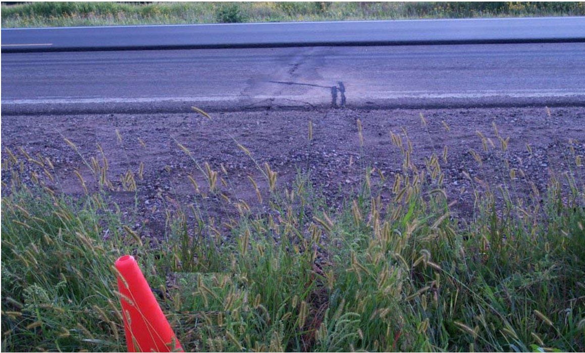
Figure 6.2. Instrumentation installation after placement of first lane.
