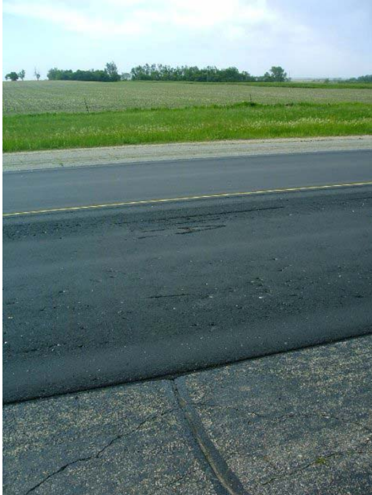
Figure 6.18. Paver-laid thin-lift overlay on US 212.
