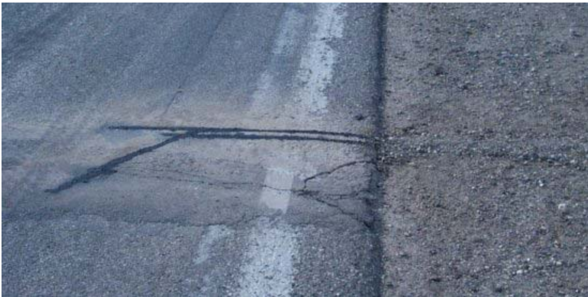
Figure 6.1. Close up photograph of thermocouple installation.
