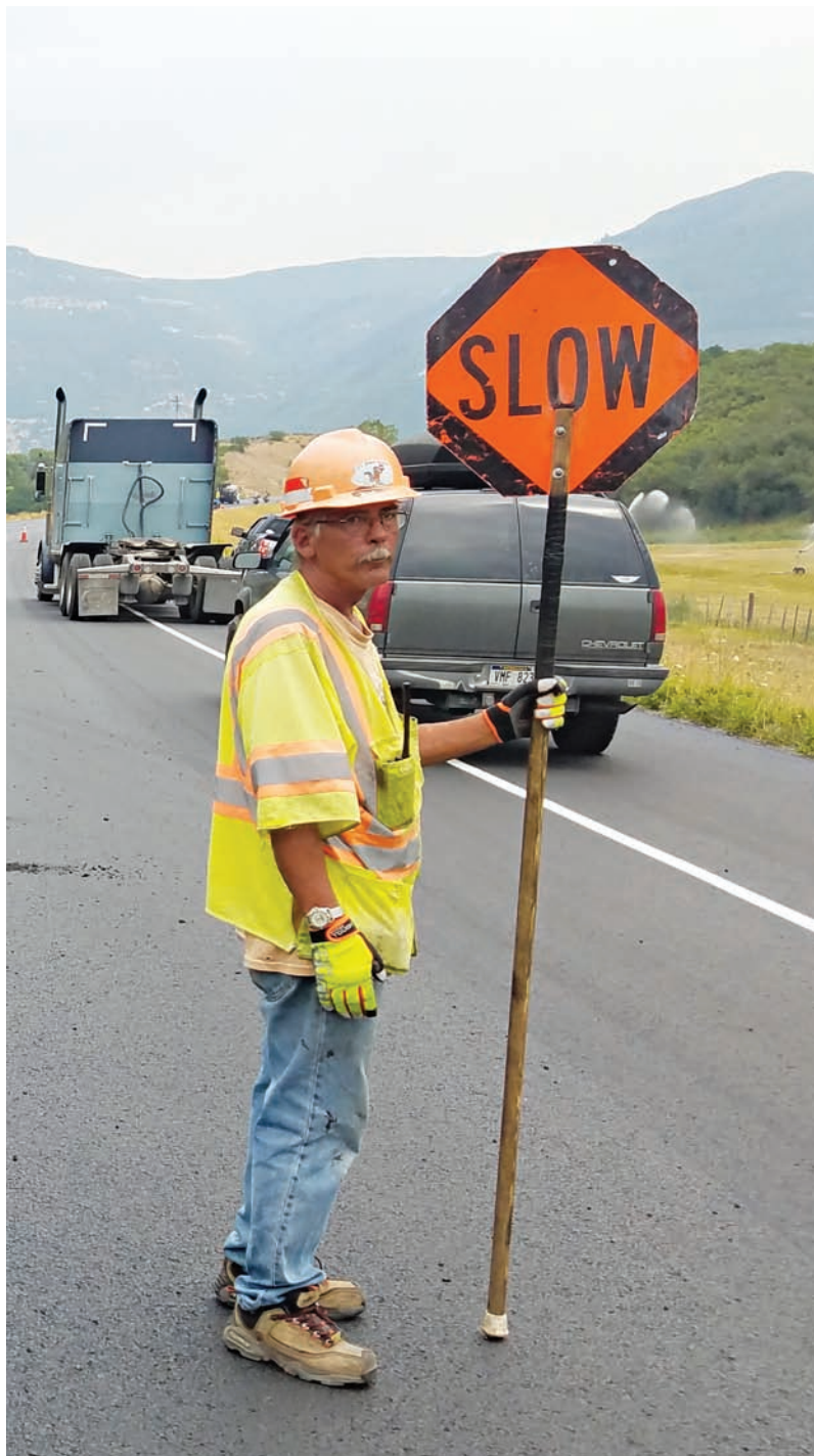
A traffic control person in the work zone with the 'AWARE' notification device on his safety vest. This works with the flagger station on either end of the project.
