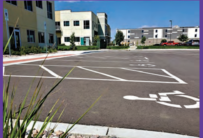
Project: 2534 Business Park (Johnstown) 85 parking spaces
