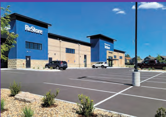
Project: Restore Retail (Colorado Springs) Paving Contractor: Martin Marietta
