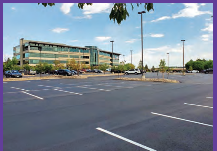
Project: ARROW Dry Creek Office Building (Denver Tech Center) 4.9 acre parking lot Paving Contractor: Denver Commercial Property Services
