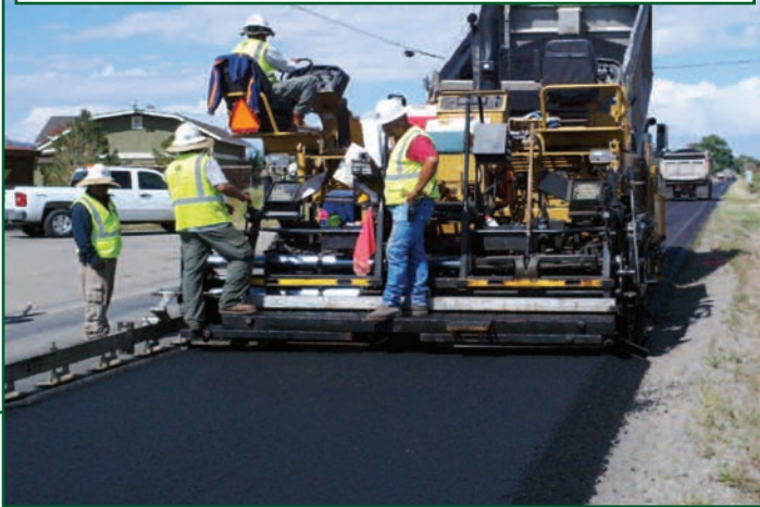
United Companies of Mesa County placing WMA on a County road.
