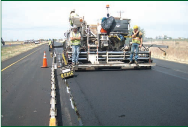
A&S Construction paves WMA on Highway 50, left. CDOT Region 2 Maintenance, right, placing warm mix asphalt on US24 on Wilkerson Pass. WMA was supplied by Lafarge West Inc. in Colorado Springs.
