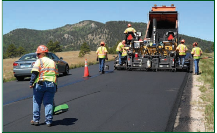
A&S Construction paves WMA on Highway 50, left. CDOT Region 2 Maintenance, right, placing warm mix asphalt on US24 on Wilkerson Pass. WMA was supplied by Lafarge West Inc. in Colorado Springs.
