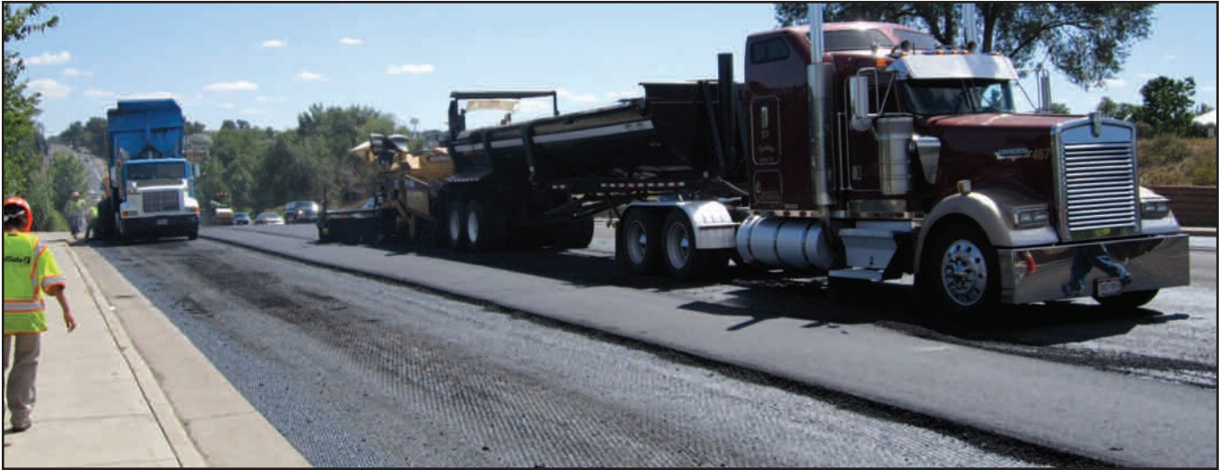
Echelon paving without interruption between project extremes minimized cold joints on CDOT's Belleview resurfacing project between Broadway and Santa Fe in Englewood. Contractor Aggregate Industries earned 100 percent of the available incentive on the project.
