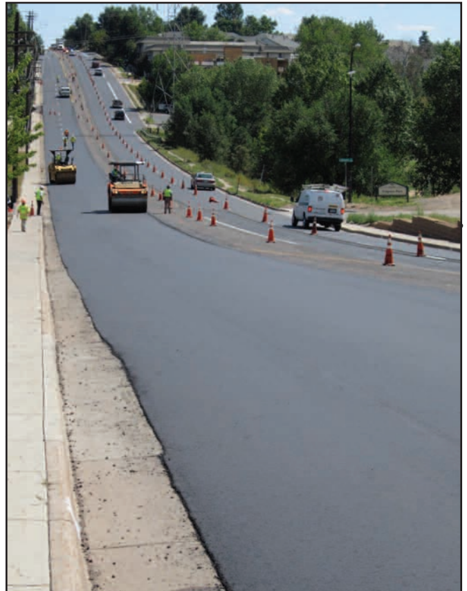
Echelon paving without interruption between project extremes minimized cold joints on CDOT's Belleview resurfacing project between Broadway and Santa Fe in Englewood. Contractor Aggregate Industries earned 100 percent of the available incentive on the project.
