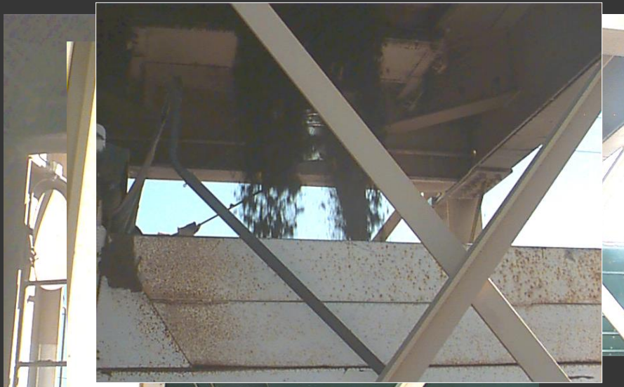
The sampler is required to pass completely through the discharge
