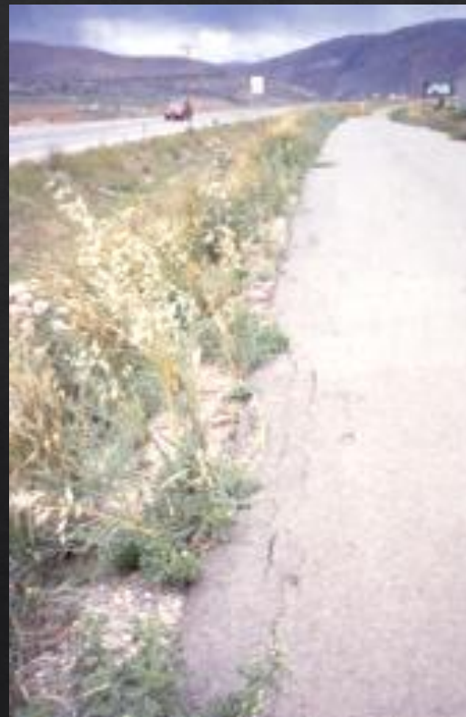
Shoulder failure
